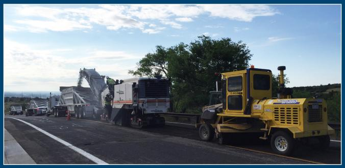
Photo 7. | Asphalt milling in progress. Photo from The City of Colorado Springs' website.
